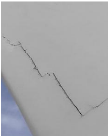
Fig.1 Blade Cracking
