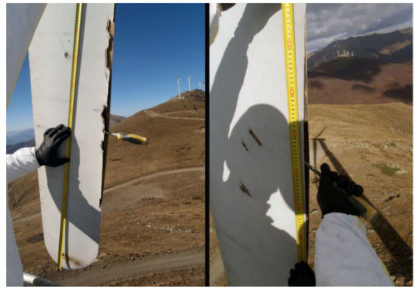
Fig.2 Fan Blade Cracking and Shedding
